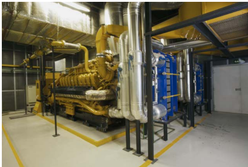
Figure 4: Four G3520C generator sets in a combined heat and power plant provide electric power, hot and chilled water to a large office complex in São Paulo, Brazil. Photo courtesy of Ecogen.
