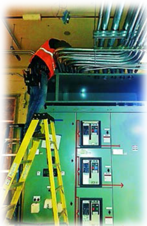
Electrician working on CAT switchgear
