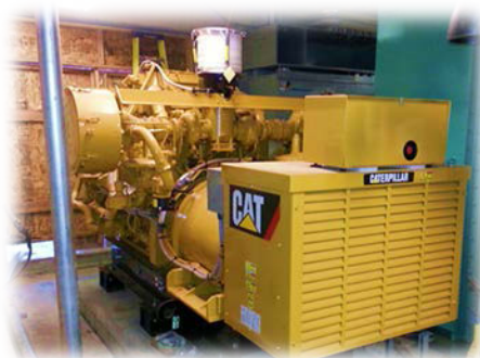
New cogen unit in place on foundation
