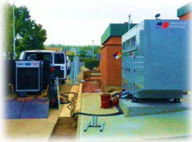
Load testing new outdoor standby genset
