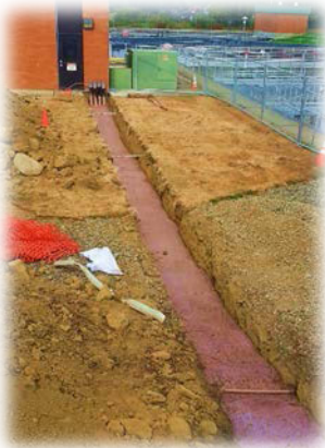
Lower portion of new electrical ductbank linking lower blower building power distribution center with cogen engine switchgear in digester control building
