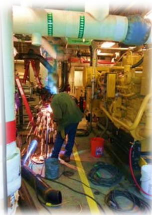
Pipefitter at work on hot water loop
