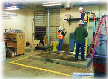
Preparing spot for new cogen unit
