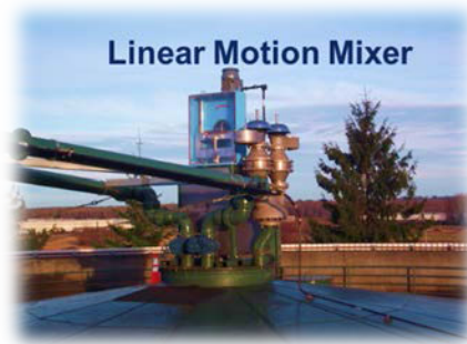
Linear motion mixers efficient mix sludge in anaerobic digesters
