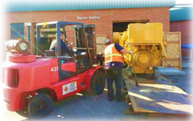
Moving new Cogen unit into digester control building
