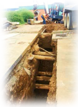
Lower portion of new electrical ductbank linking lower blower building power distribution center with cogen engine switchgear in digester control building
